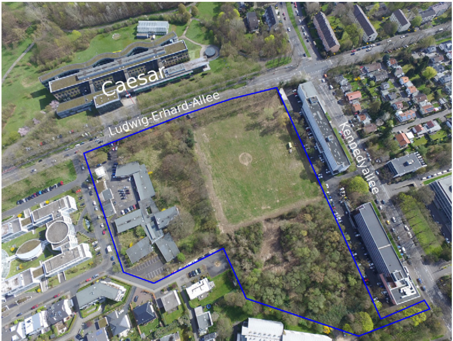
Planning area for the new building of the BSI
